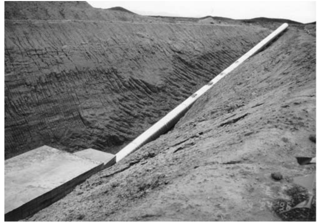
FIG. 19. The PALO VERDE underground laboratory at the time of construction (fall 1996).
