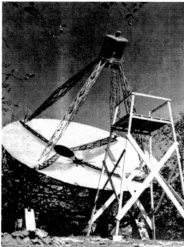
FIG. 8. Grote Reber's radio telescope at his home in Wheaton, Illinois, circa 1939. Reproduced courtesy of G. Reber.
