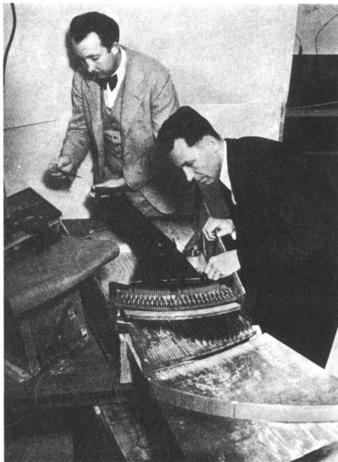
FIG. 21. General view of multicrystal spectrograph with cover of lead enclosing box removed. The baffles for reducing the fogging caused by diffuse scattering can be clearly seen as can also the curved graphite scattering body in the foreground.
