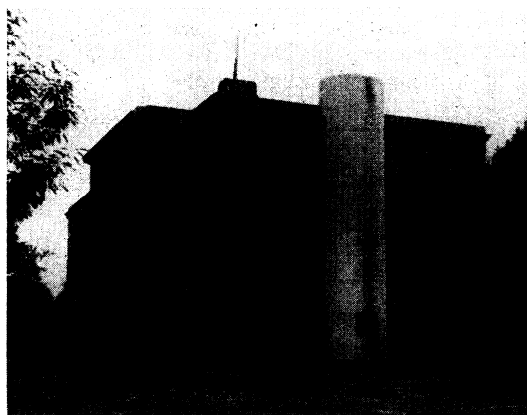
FIG. 8. Tank in which apparatus is installed. The upper part is filled with water. The apparatus is in the lowest 12-ft. section.
