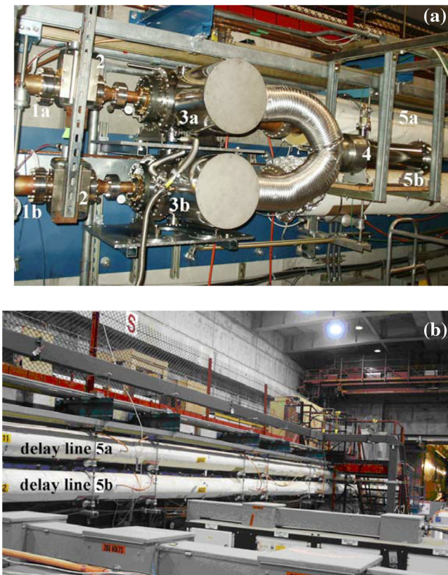
FIG. 7. General view of two-channel active SLED-II pulse compressor: (a) 1a,b—top and lower input waveguides (operating at the mode TE_{01} ); 2—ion pump; 3a,b—top and lower plasma switches; 4—high-voltage generator; 5a,b—top and bottom storage delay line. (b) Top and lower storage delay line.
