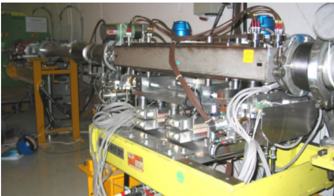
FIG. 3. (Color) The installation of the prototype LHC collimator in the SPS tunnel. The figure is taken from [31].
