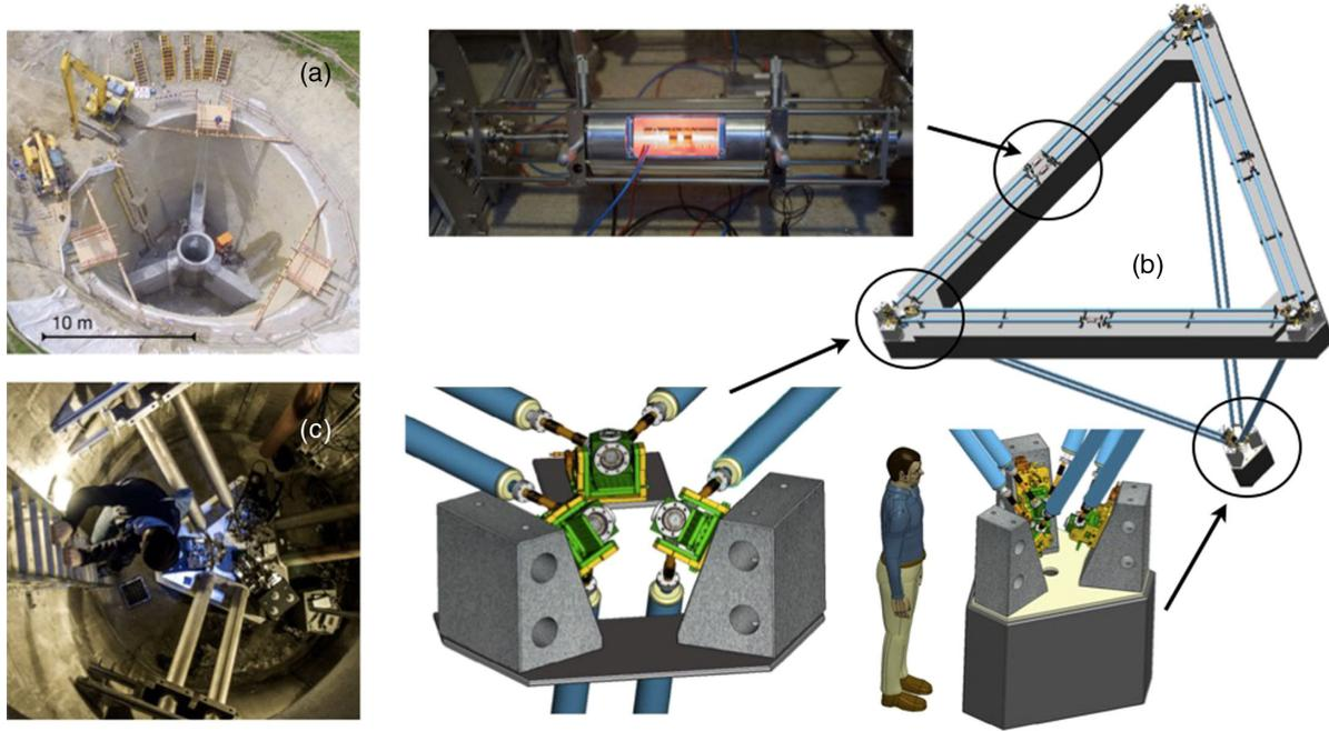
FIG. 1. Construction site of the four-component ring laser structure at the Geophysical Observatory, Fürstentfeldbruck (near Munich, Germany). The excavated location for the monument of the optical resonator (a) provides the room for the tetrahedral gyroscope layout (b). The apex at the bottom of the monument (c) is rigidly attached to the triangular concrete frame on the top by a massive concrete support structure.
