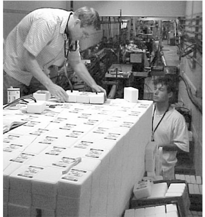
FIG. 5. View of the salt stack construction at the antenna layer. Antennas were mounted with their leads passing through drilled salt blocks as seen in several examples on the top of the stack.
