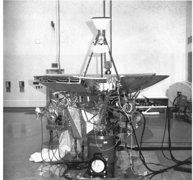
FIG. 1. NASA photo No. 72HC94, with caption “The Pioneer F spacecraft during a checkout with the launch vehicle third stage at Cape Kennedy.” Pioneer F became Pioneer 10.
