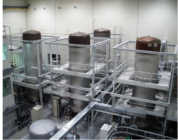
FIG. 3. Photo of some Virgo mirror UHV chambers.
