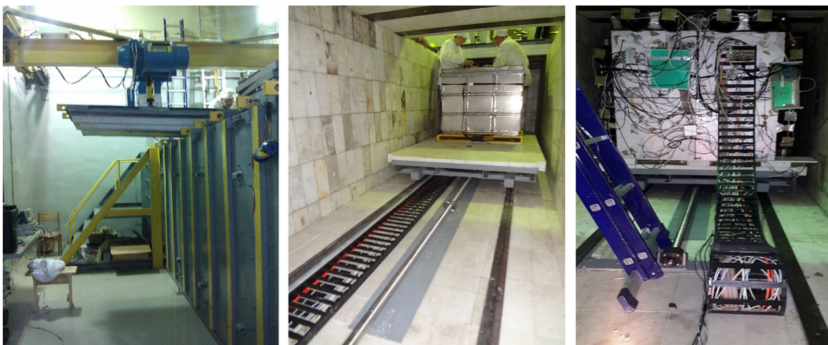
FIG. 3. General view of passive shielding: from the outside and inside. The range of detector movements is 6–12 m from the center of the reactor core on the left. Model detector is in the center; full-scale detector is on the right.
