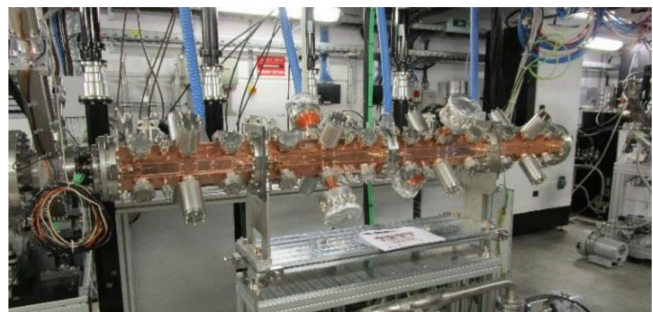
FIG. 3. Installation of the radio frequency quadrupole of the LIGHT prototype in the bunker test area in 2017.
