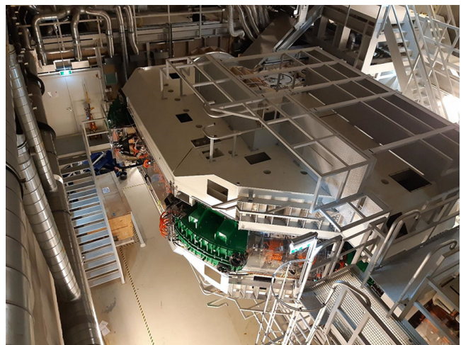
FIG. 7. Bird view look at the MedAustron gantry laying in the horizontal position (gantry rotation angle 90°). The gantry entrance is in the lower-right corner of the picture.
