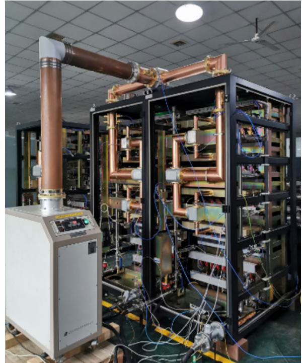
FIG. 26. Test setup of the 50-kW power amplifier.
