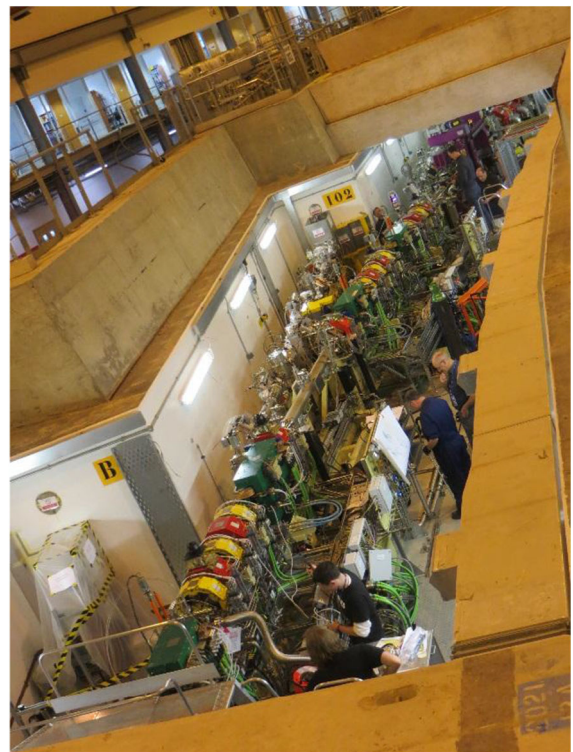
FIG. 12. DDBA girders installed in the tunnel.
