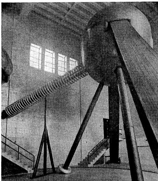
FIG. 1. View of 1.8-Mv generator and accelerating tube.
