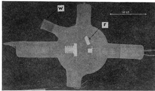
FIG. 2. Photograph of x-ray tube.
