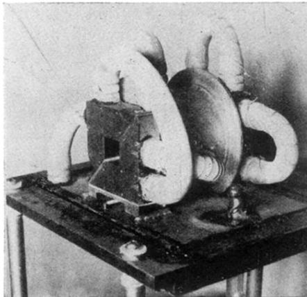
Fig. 1. Photograph of the tungsten furnace.
